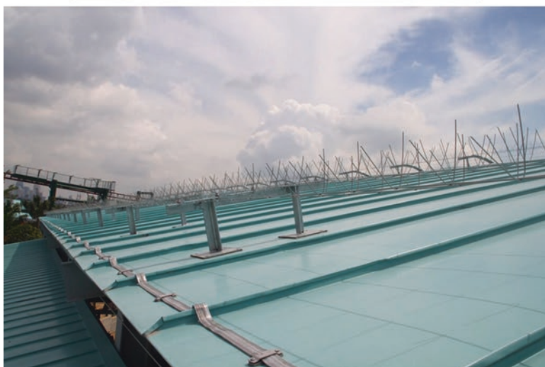
Fig. 17.6 “Lightning eliminators” – not accepted by any lightning standard. (Courtesy of HCFP Pte. Ltd.)
