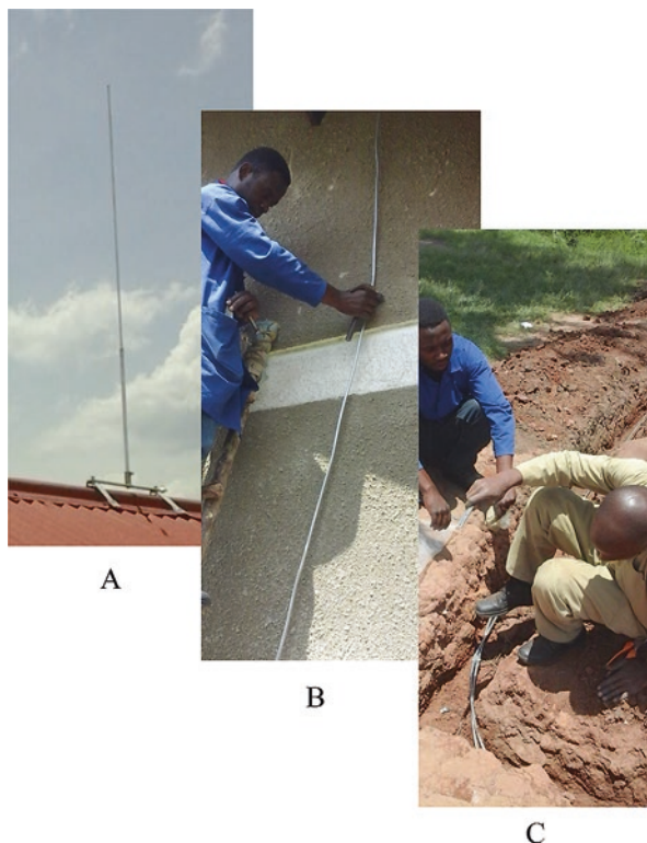
Fig. 17.1 Installation of (a) air terminal, (b) down conductor, and (c) ground terminal at school in Uganda. (Courtesy of ACLENet)
