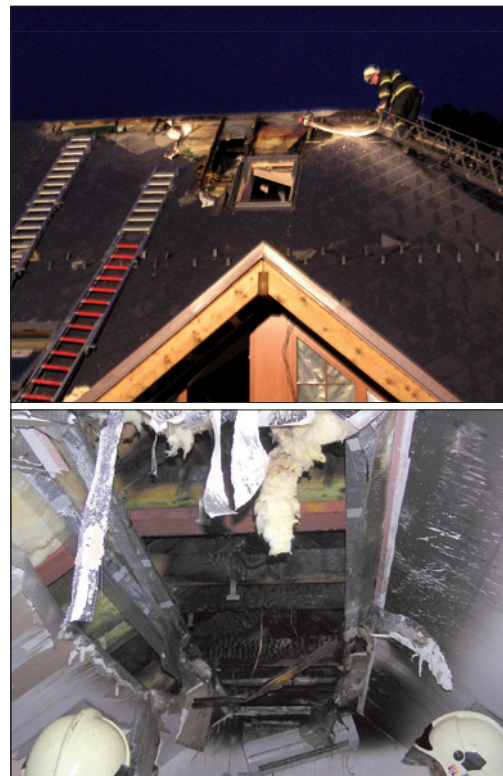
Fig. 2 Burning-in of the hotel's attic
