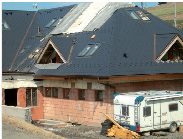
Fig. 6 Situation after extinguishing fire
