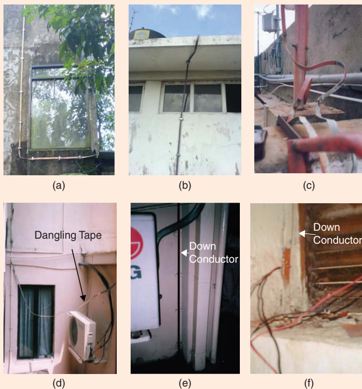
Fig. 3. Erroneous installation of down conductors. a) Right-angled bend about 3-m above ground level. b) U bend close to windows. c) Crooked and twisted down conductor. d) Loosely hanging part of a down conductor. e) Down conductor running very close to an entrance and to electrical equipment (down conductor is highlighted by a black line). f) Down conductor where the ground termination cannot be traced.
