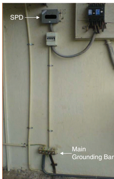
Fig. 4. Misunderstanding of standards. The technical personnel who designed this installation successfully achieved (as he understood) less than 50-cm tape length between the main grounding bar and the earth. The incorrect positioning of the main grounding bar makes the wire length between the SPD and the main grounding bar more than 2 m, which is a Standards violation [15]. At such a location with no space restriction the designer could have easily planned the positions of both the SPD and the main grounding bar to be well in compliance with the recommendations of [15].
