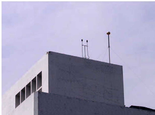
Fig. (7). Lightning strike to a point within 10 m of a Dynasphere placed in accordance with the CVM [19].
