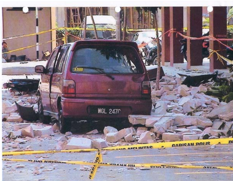
Fig. 3. Fallen rock from struck building – hazard arising from invalid ESE/CVM theories.
