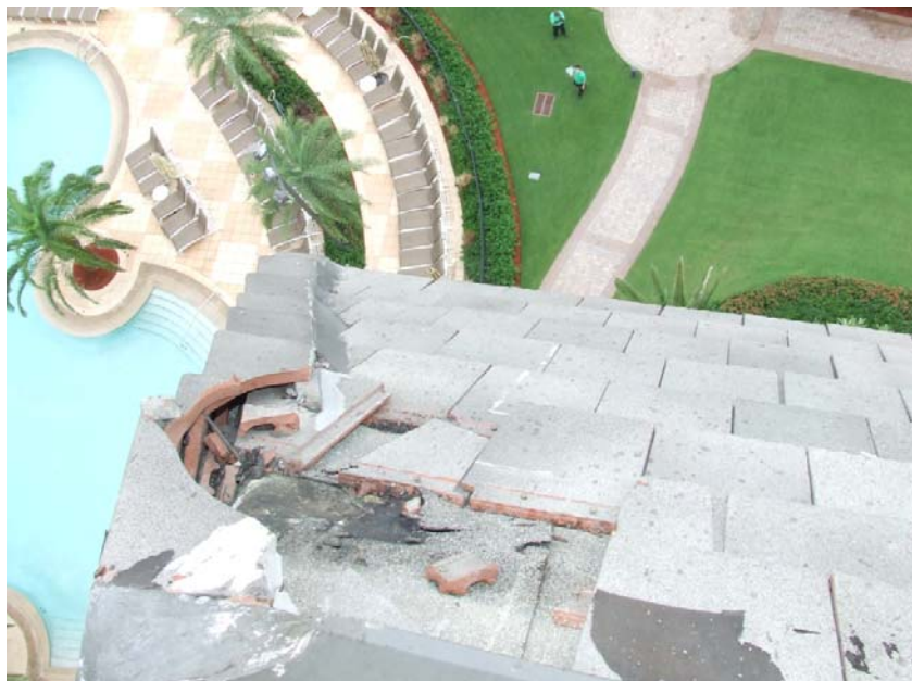
Fig. 4. ESE failure incident at Maripott Hotel in Marco Island, Florida [25.1].
